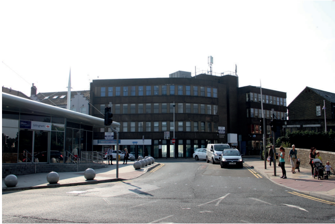
Railway station, High Street (far east)
