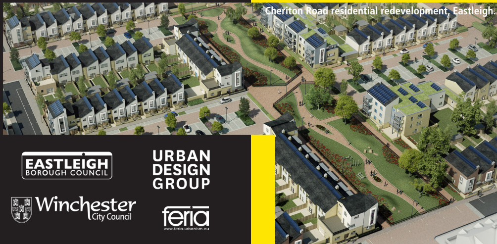
Cheriton Road residential redevelopment, Eastleigh.
