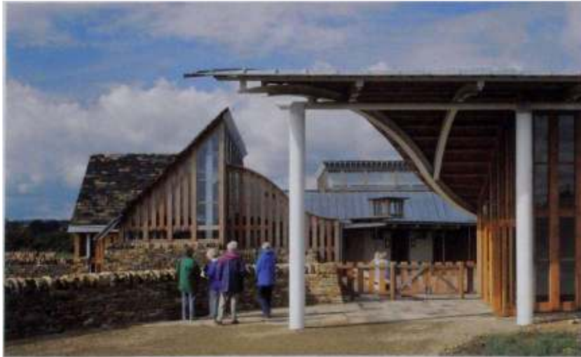
Left: Fountains Abbey Visitors Centre, North Yorkshire. The use of traditional and modern materials to create distinct building forms that blend
